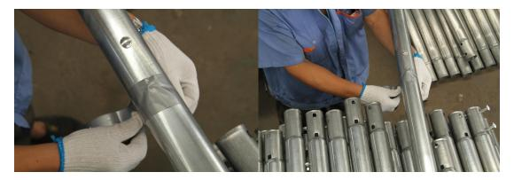
Please use the tape wrapped around the gap between the steel skeleton after installing.
